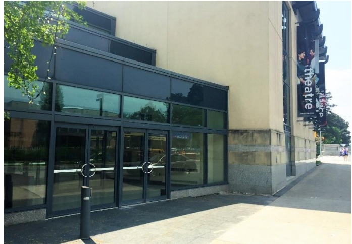
The soon-to-be North York Arts entrance, facing North York Blvd.
