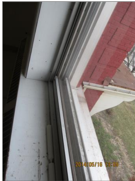
Example of the original double hung windows and evidence of condensation deteriorating the wood window sill.
