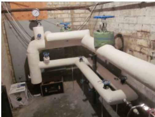
Figure 3.1: Main Steam Pipe
