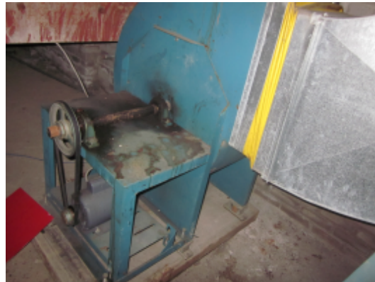
Figure 3.9: Washroom Exhaust Fan
