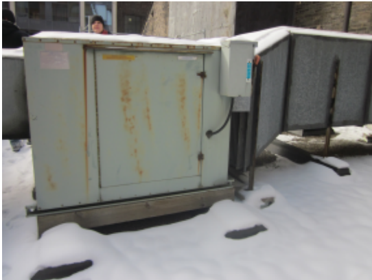
Figure 3.8: General Exhaust Fan
