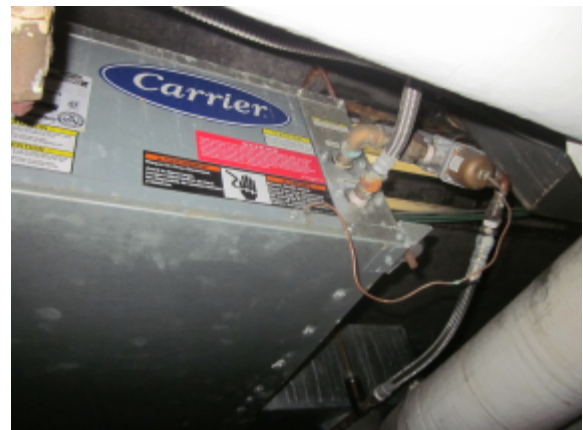
Figure 3.7: Heat Pump
