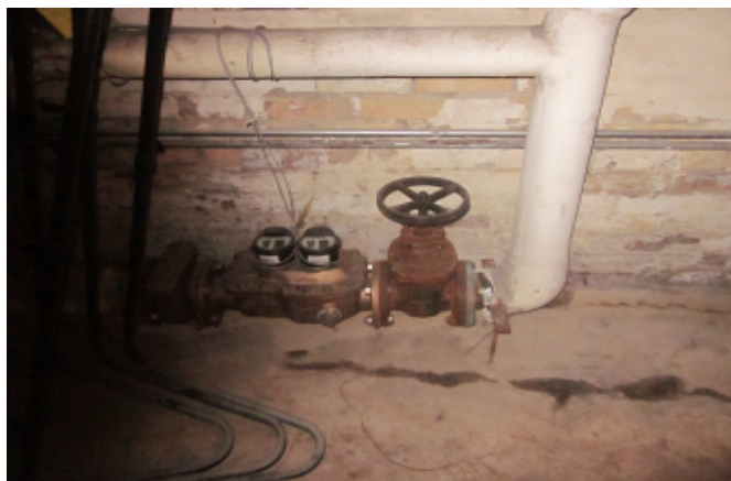
Figure 3.12: Water meters
