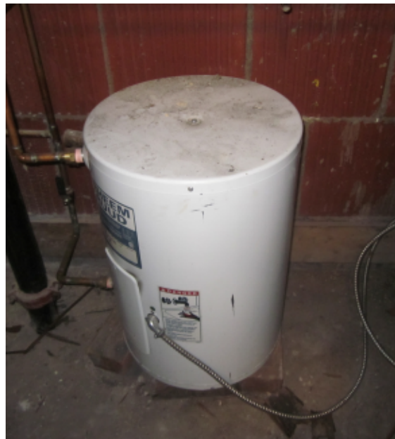
Figure 3.16: Electrical DHW heater in right balcony closet
