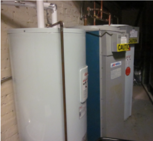
Figure 3.13: Electrical DHW heaters
