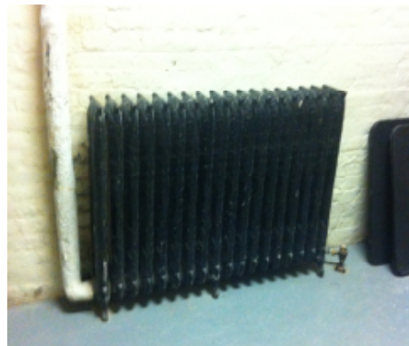
Figure 3.2: Perimeter Steam Radiator
