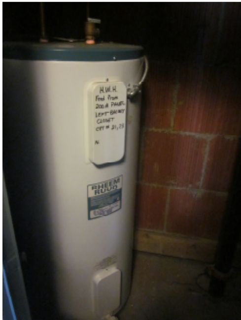
Figure 3.15: Electrical DHW heater in left balcony closet
