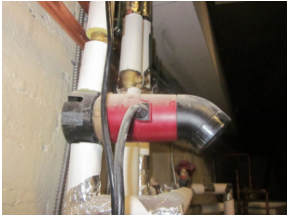
Figure 3.14: DHW recirculation pump
