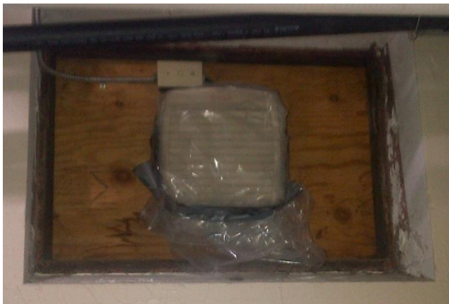
Figure 14: Exhaust fan installed in Theatre basement window.
